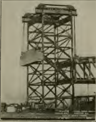
VIEW OF SOUTH TOWER.
